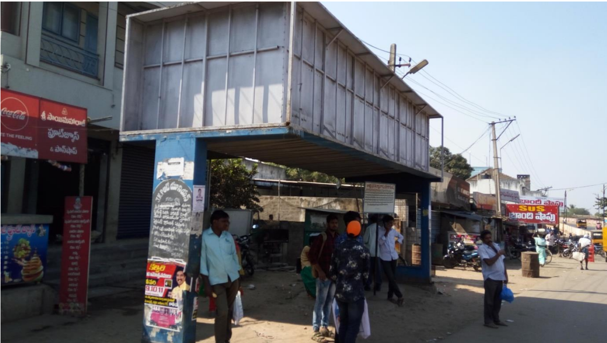
Figure 11 Bus Shelter at J.G.puram ( Ramchandrapuram Side)
