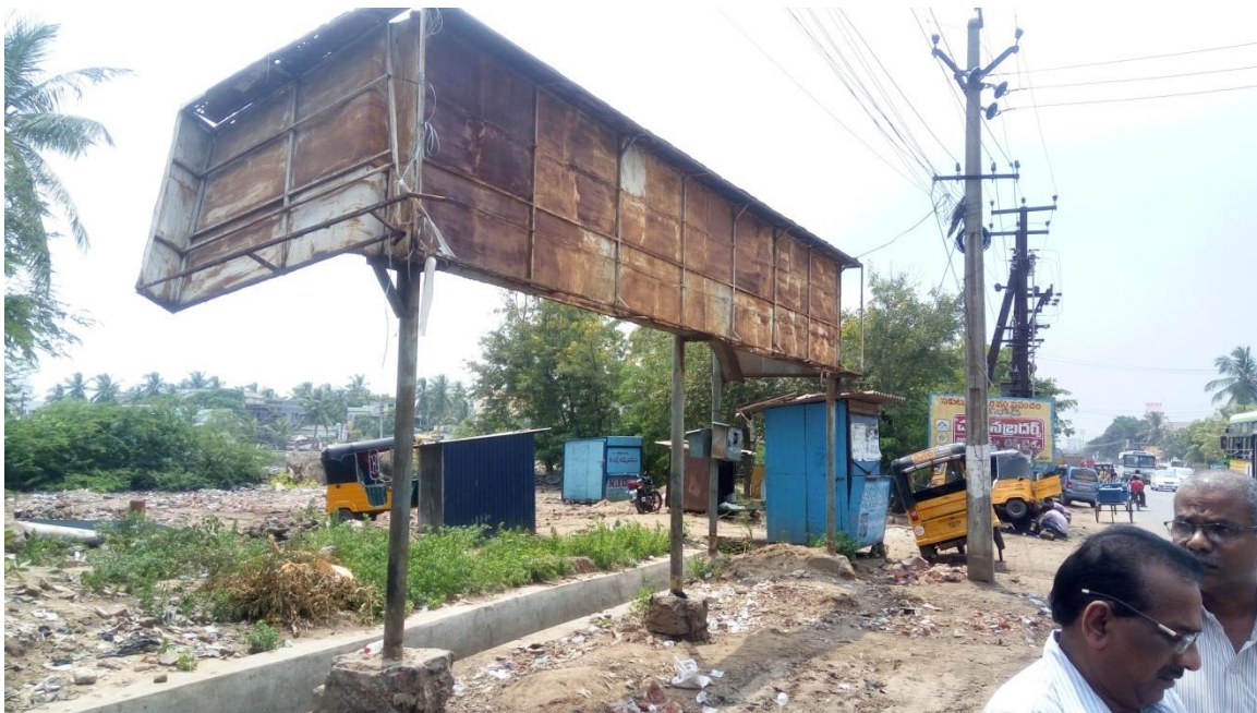
Figure 4 Bus Shelter at Annam Ghati
